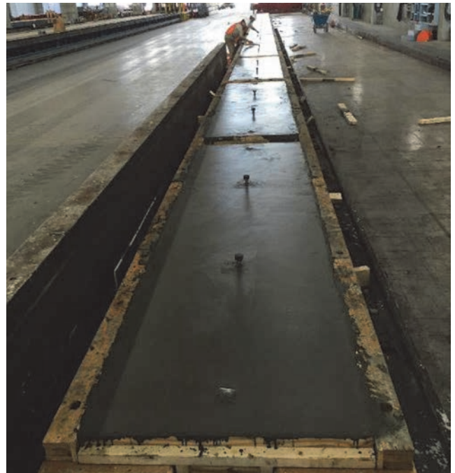
Figure 11. Beam specimens after casting of concrete
