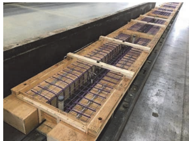
Figure 8. Form after placing reinforcement
