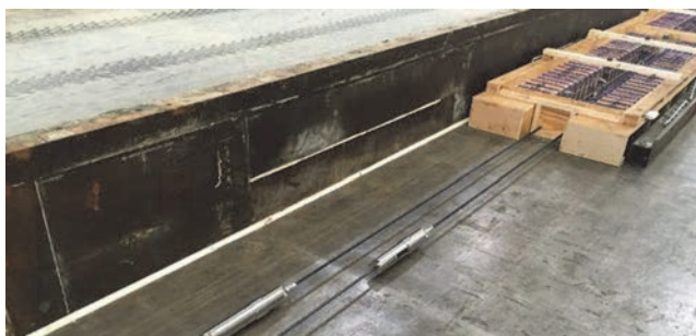
Figure 10. CFCC strands after tensioning
