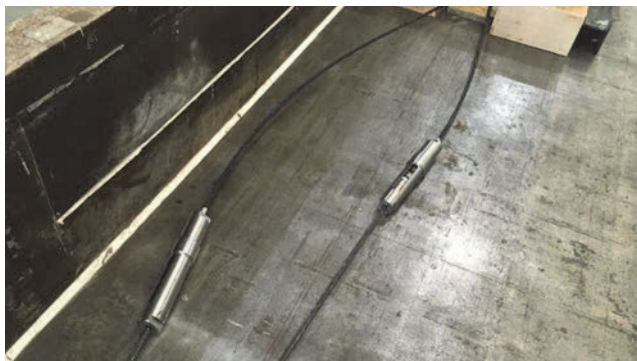
Figure 9. CFCC strands before tensioning
